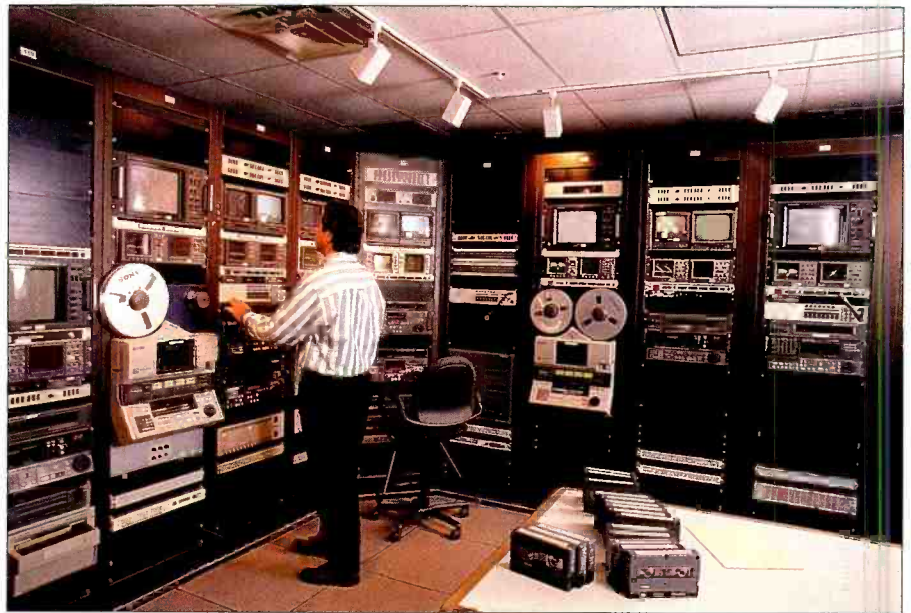
The tape operations area where machines of various tape formats are available for dubbing and on-air operations.
