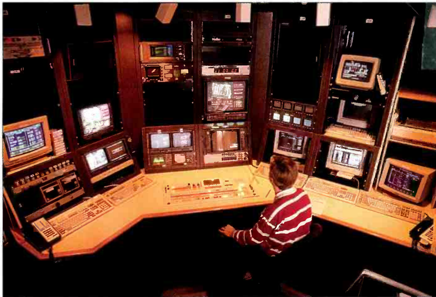
The master control area at KHOU-TV. Despite using switches that allow a single keyboard to be used with several computers, keyboards tie up considerable desktop workspace.
