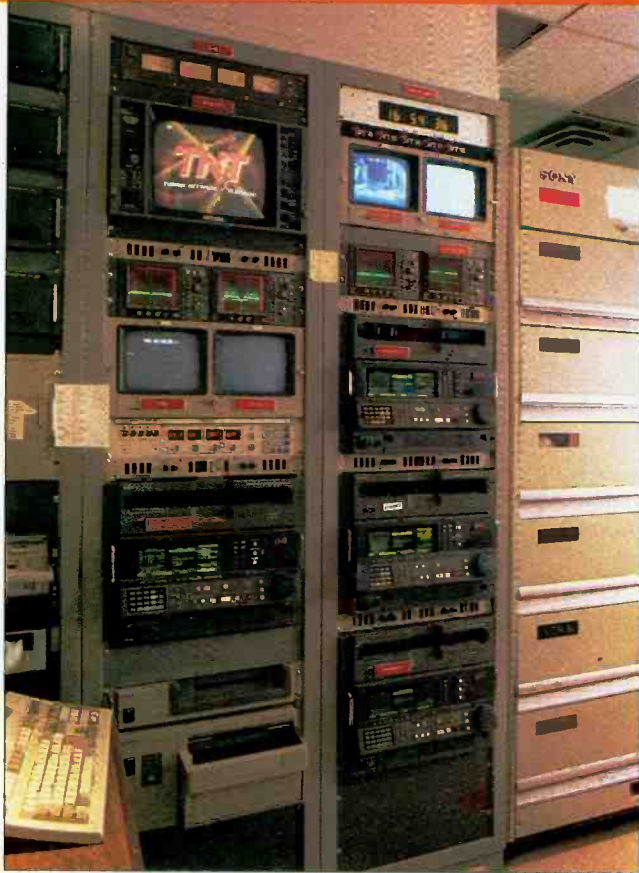
External VTRs under cart machine control at TNT Latin America.
