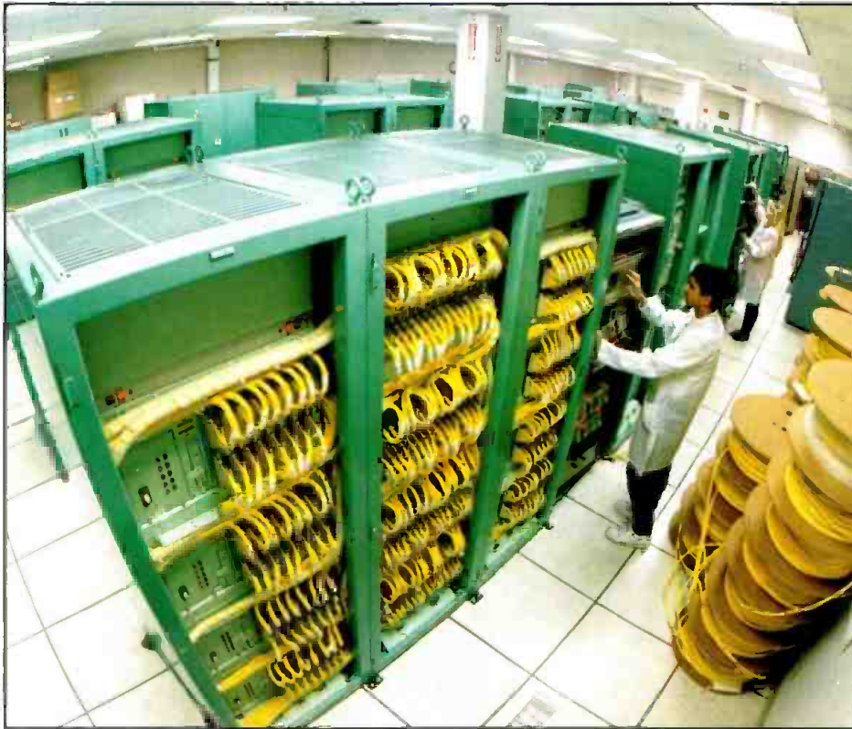
A 512 x 512 digital switcher incorporating fiber-optic I/O and operating at up to 1.2Gbit/s rates. (Courtesy of TRW.)
