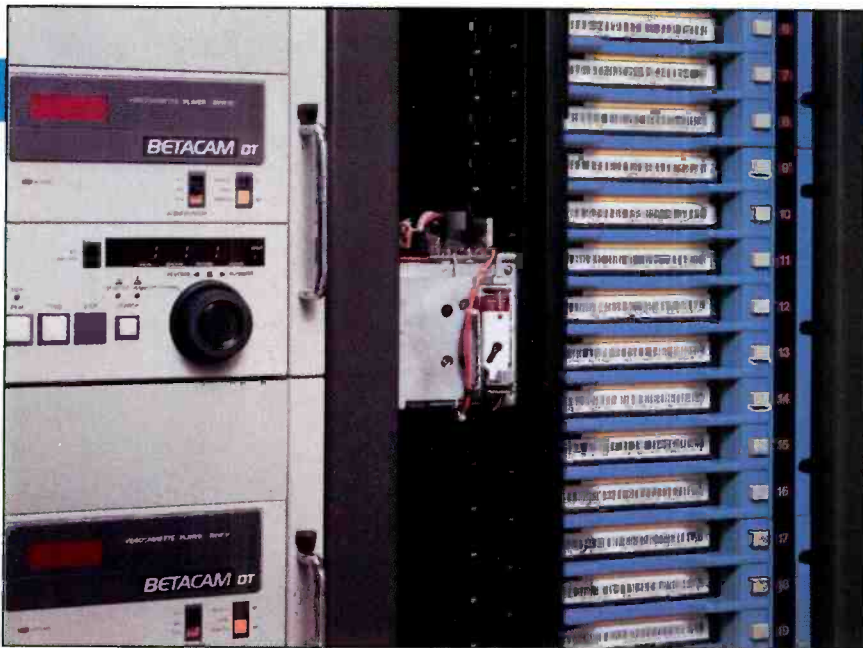
This robotic elevator moves vertically in the space between the storage bins and the side-loading tape machines. A bar code reader in the elevator identifies the tape, which is marked by a bar code label pasted to the back edge of the cassette housing.
