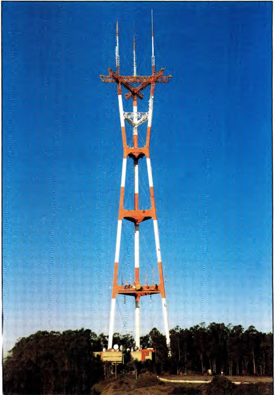
The shared transmission facility on Mount Sutro in the middle of San Francisco came through the earthquake in perfect shape. Built on bedrock, the 977-foot tower and its arrays are designed to withstand a quake measuring at least 8.3 on the Richter scale. During the quake, the tower moved, but stayed well within its design parameters. (Photo by Don Lincoln, Sutro Tower.)
