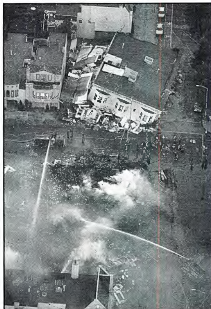
Bay Area broadcasters were spared the kind of damage the quake inflicted on the Marina District near the Golden Gate Bridge. Unlike the bridge, the Marina is built entirely on bay fill, which went into liquefaction during the shaking, amplifying ground movement. Gas pipes ruptured and exploded as buildings crumbled. With pressure down to fight fires, only water pumped from the nearby San Francisco Bay prevented tragedy from becoming catastrophe. (Photo by Deanne Fitzmaurice, San Francisco Chronicle.)
