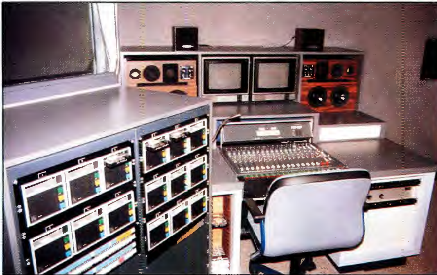
Cartridge machines have become a key component in both on-air and production work. Despite the progress made by digital storage systems, the cart machine remains the primary source of commercial and music playback.
