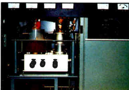
One of the Klystrode tube visual amplifiers in operation at WCES-TV, channel 20 in Wrens, GA. The double-tuned output cavity can be seen in the center of the photo.
