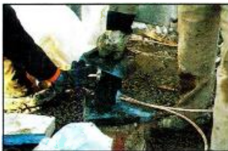
Cadwelding is the preferred method of joining elements of a ground system. This photo sequence illustrates the procedure. Photo (a) shows the powdered copper oxide and aluminum compound being added to the Cadweld mold after the conductors have been mechanically joined. Photo (b) shows final preparation of the bond before igniting. Photo (c) shows the chemical reaction that produces the excellent bond provided by Cadwelding.
