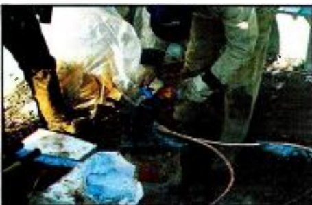
Cadwelding is the preferred method of joining elements of a ground system. This photo sequence illustrates the procedure. Photo (a) shows the powdered copper oxide and aluminum compound being added to the Cadweld mold after the conductors have been mechanically joined. Photo (b) shows final preparation of the bond before igniting. Photo (c) shows the chemical reaction that produces the excellent bond provided by Cadwelding.
