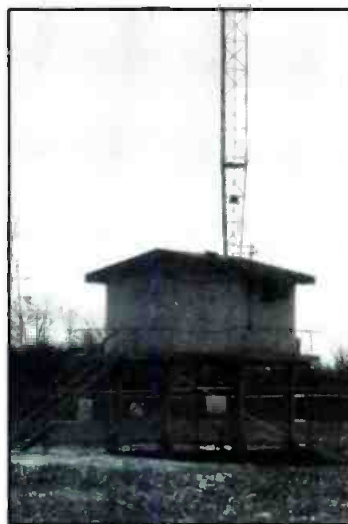
A Continental 1 kW AM transmitter installation for KPBC in Dallas.
