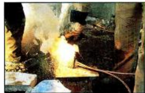
Cadwelding is the preferred method of joining elements of a ground system. This photo sequence illustrates the procedure. Photo (a) shows the powdered copper oxide and aluminum compound being added to the Cadweld mold after the conductors have been mechanically joined. Photo (b) shows final preparation of the bond before igniting. Photo (c) shows the chemical reaction that produces the excellent bond provided by Cadwelding.
