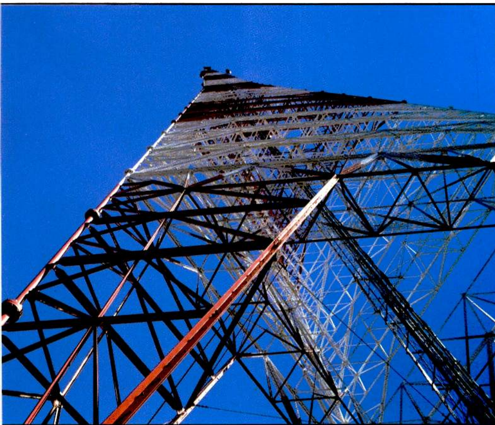
The 1,067-foot WNEV-TV tower, Newton, MA, is a prime candidate for heavy winter icing.
