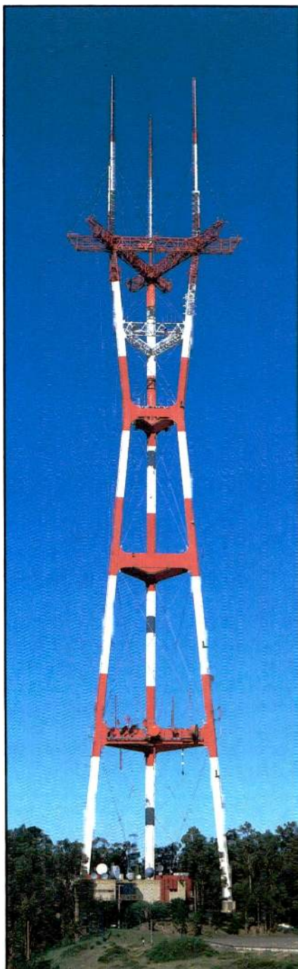
Sutro Tower is a landmark in San Francisco and is familiar to broadcast engineers throughout the country.
