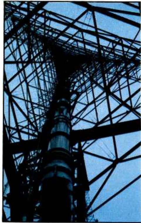
Cross-bracing in the tower for KTZZ-TV 22 (Seattle) adds structural strength to faces and the cross-section.
