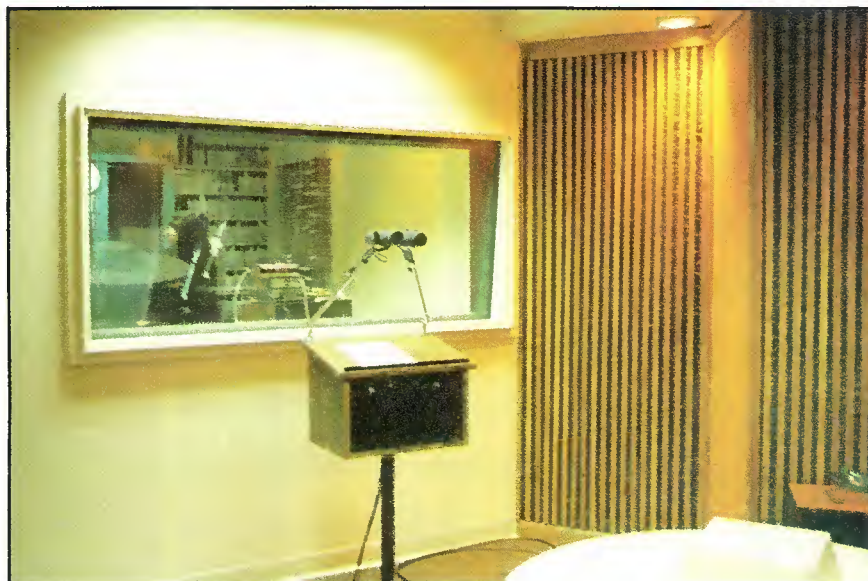
This interior view of a production studio shows splayed walls with panels of fabric-faced absorption alternating with absorption faced with wood battens.
