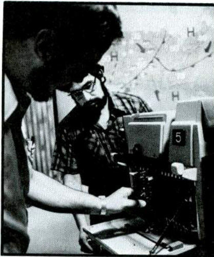
Boards are easy to access, but service has not been needed thus far.
