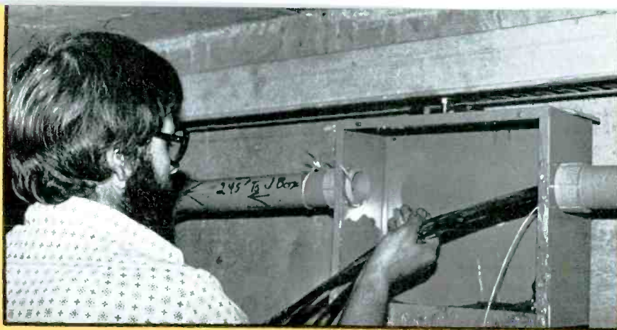
A Great Lakes Electric technician feeds cables into conduit.
