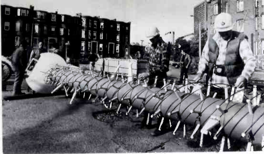
Cetec Jampro technicians inspect Spiral antenna bay prior to airlift. Sections were trucked from Sacramento to Boston.
