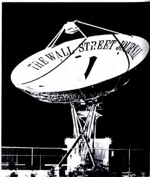
The Wall Street Journal's 4.5-meter (15-foot) receive-earth station located near Kissimmee, Florida. (Photo courtesy of Western Union.)
