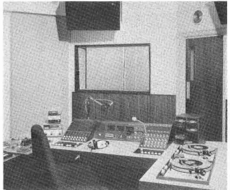
Fig. 9 A western station? No, but it could be. This layout is not so unique. What is different is the unique control board. It's currently in use at Piccadilly Radio, London. We included it here because it makes use of the slide controls which are coming into fashion in current board design. (Photo courtesy of Rupert Neve)
