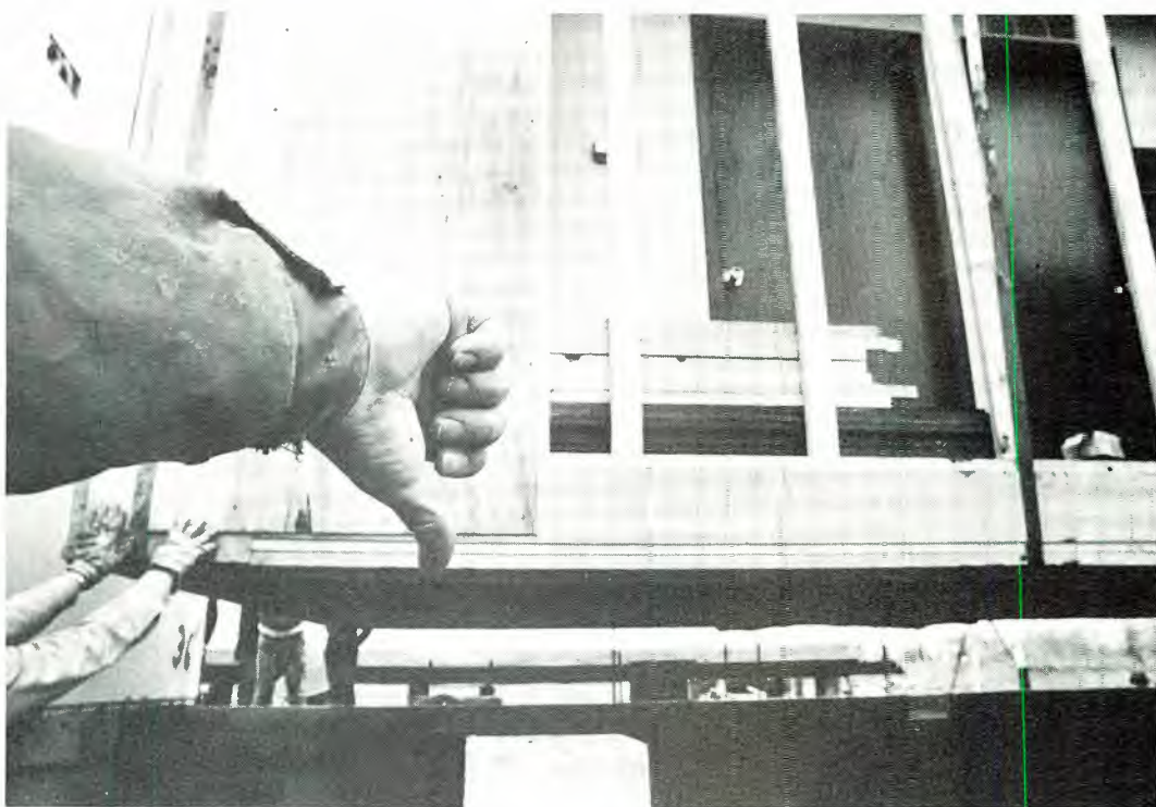
Fig. 2 As you can see in the detail of this picture, the WFMS structure was pre-built inside the SAI factory before being hauled to the new site. Note that the doors are already hung, and even the thermostat is wired in.
