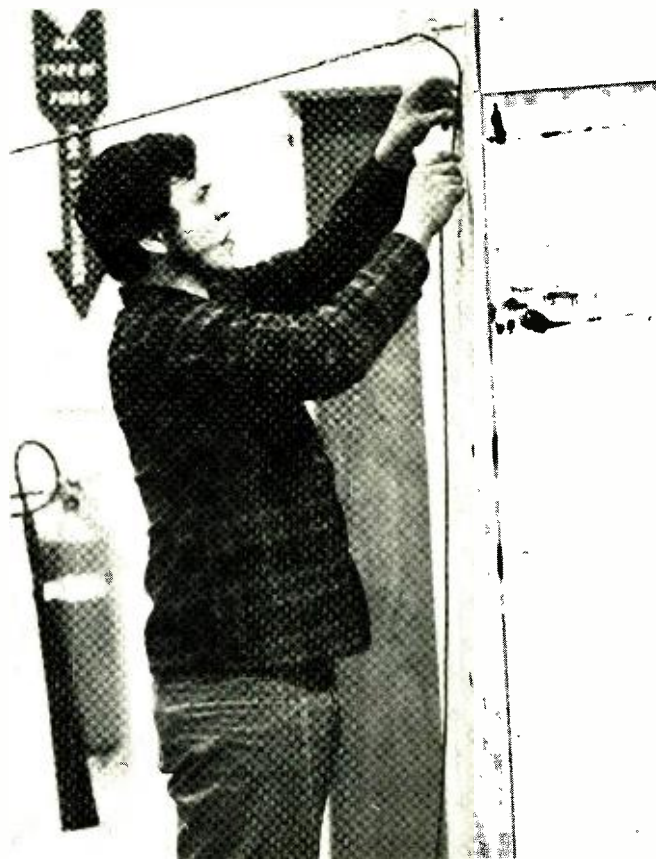
Fig. 2 Victor Miranda of National Trans Video, Los Angeles, practices installing drop cable.
