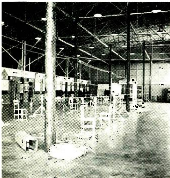
Fig. 1 Inside training area at Texas A&M showing poles and strand ready for practice installation. Hanger is shared with telephone and power lineman training schools.
