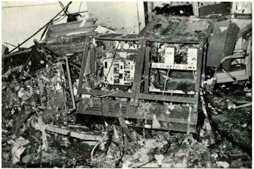
Fig. 4. WLOX-TV after the water receded. Barely recognizable equipment was buried under debris and mud.
