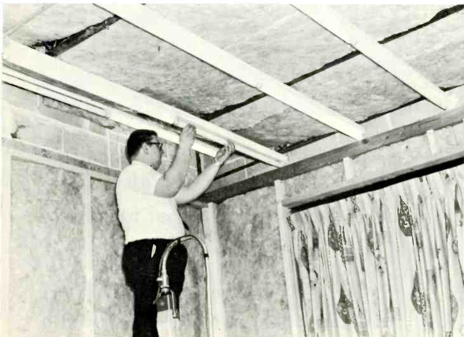
Fig. 6 View of construction details before custom walls and ceiling were installed.
