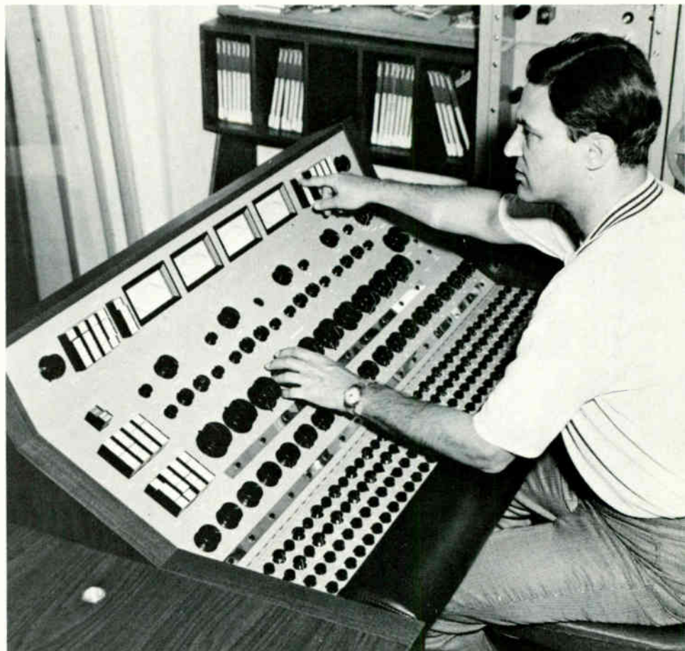
Fig. 1. Operator at main operating panel. Note subpanel arm rest.
