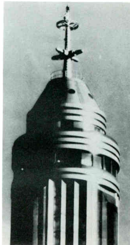
Fig. 2. 1939-1946 antenna had visual (lower) and aural (upper) elements.
