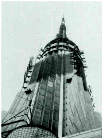
Fig. 4. "Yagi" arrays are for ch 13.
