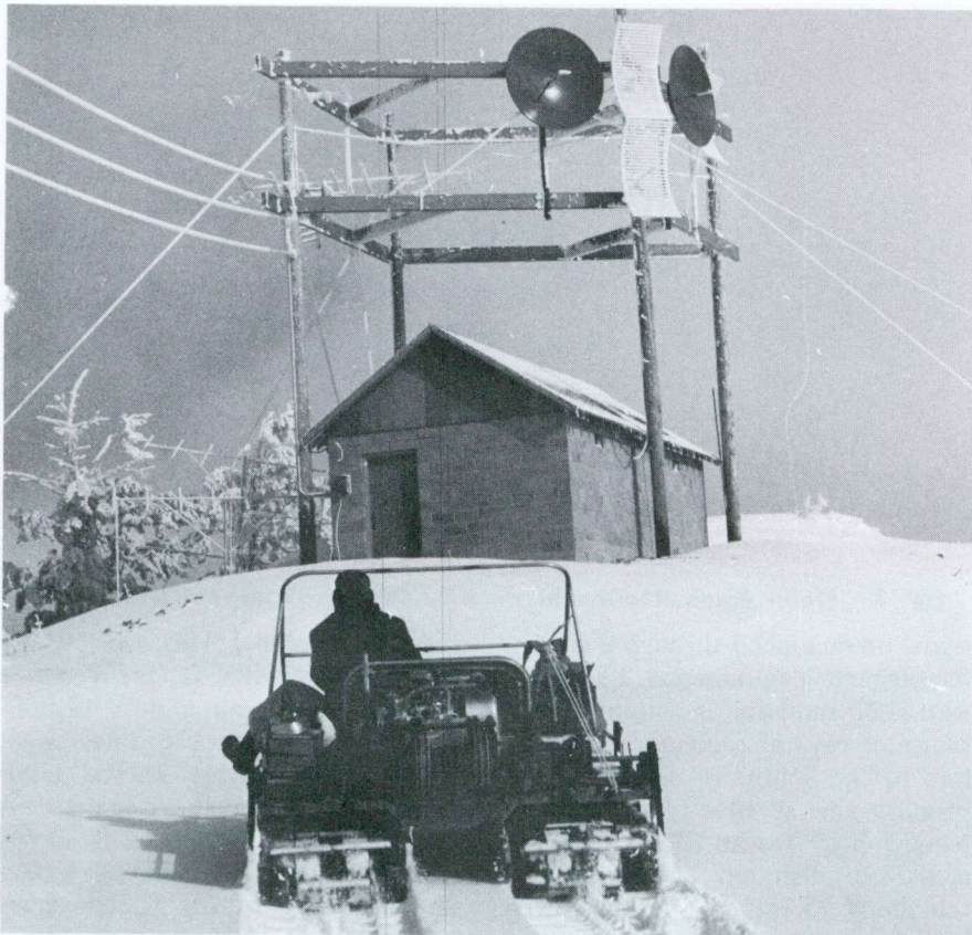
Fig. 4. Levan site shows winter maintenance facilitated with use of snowcats.
