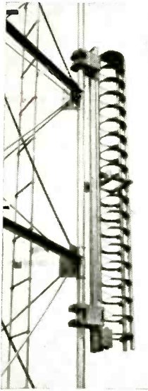
VHF-TV Transmitting Antennas
