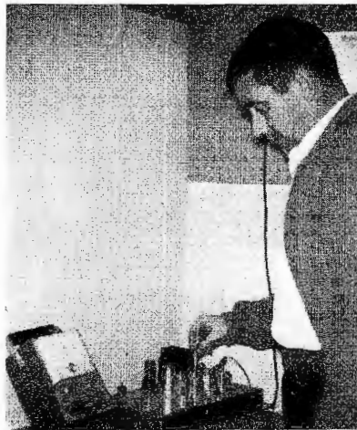
Fig. 3. Technician adjusting SCA receiver discriminator at the customer's location.
