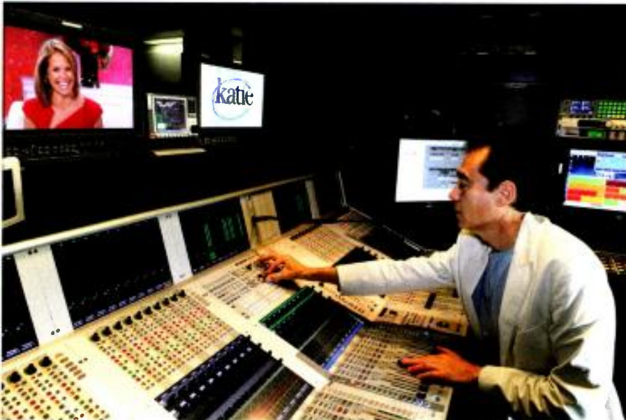
A 60-fader Studer Vista 9 audio console, supported by two Soundcraft mixers, serves the show’s needs, including supporting appearances by live musical acts. Recent acts have used rental equipment that includes Riedel RockNet interfaces.
