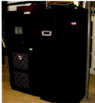
The slim footprint of the VDC flywheel is easy to pair with three-phase UPS systems.
