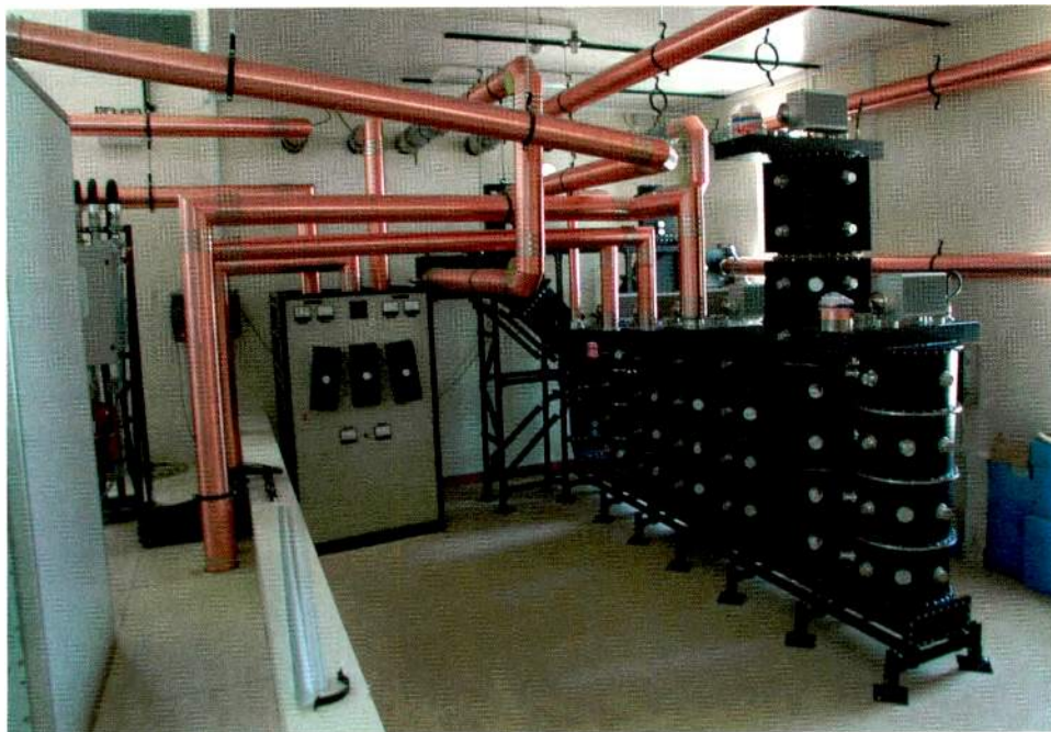
In indoor applications, where tight spaces mean tight bends, unflanged rigid line comes into its own.
