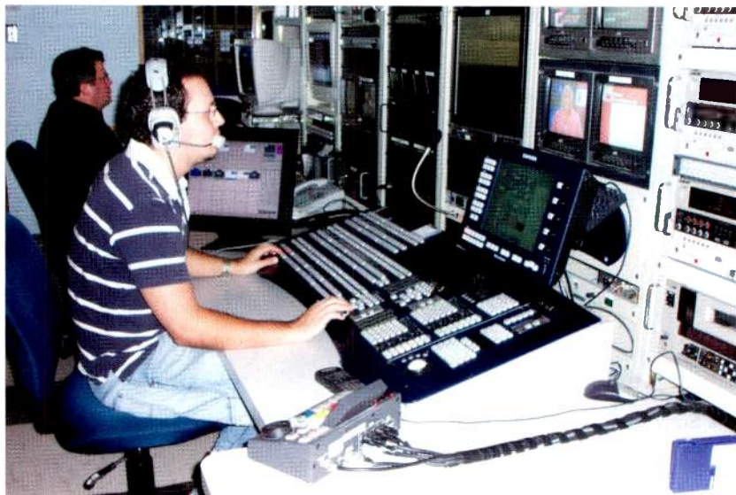
Brian Prom, director at KEYC-TV in Mankato, MN, uses a Snell & Wilcox Kahuna multiformat SD/HD production switcher in the station's control room.
