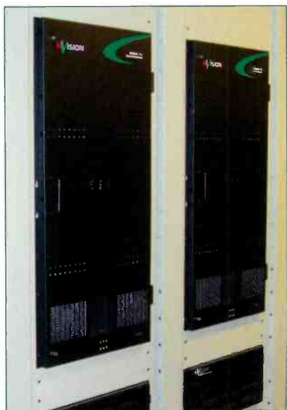
The LDS Church Conference Center in Salt Lake City uses two interconnected NVISION 8256-Plus 256x256 expandable video routers.
