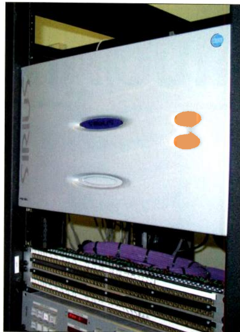
Routers, like this one from Pro-Bel, offer the ability to handle analog and digital audio as one interconnected standard.
