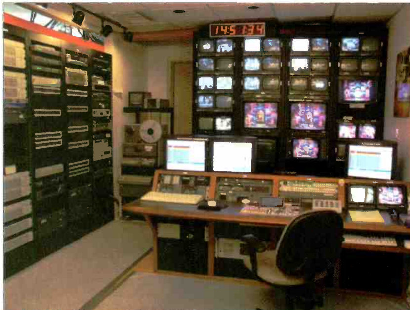
DST replaced KBWB's analog master control with a new digital center capable of multichannel streaming. The station chose an automated on-air delivery system to reduce its operational costs while establishing a clear signal path for the three channels.
