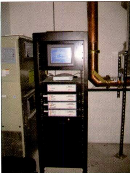
The proposed monitoring system uses a ZTechnology DM1010W professional ATSC/8-VSB demodulator and a proprietary, menu-driven, PC-based Visual Basic program.
