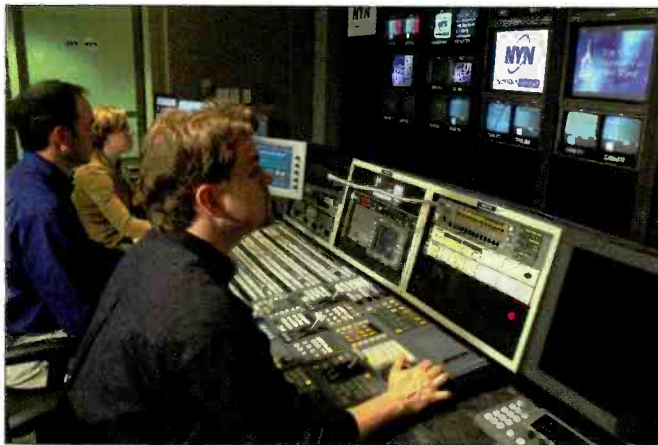
A New York Network engineer works at the Sony MVS-8000 multiformat switcher with integrated digital multi-effects.
