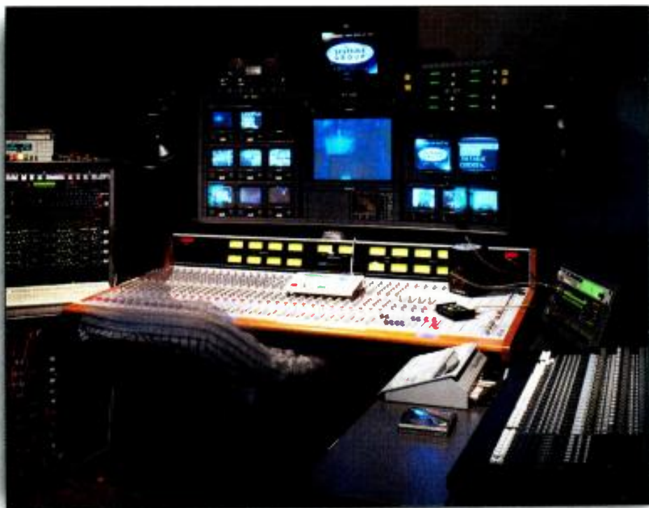
The Audio Control Room has a Wheatstone SP8 32x4x2 mixing console, ProTools 24 mix plus, Sony dual diversity WRR 840A UHF receivers, Tascam 40 MK II DAT, and 360 Systems 2730 Digicart.
