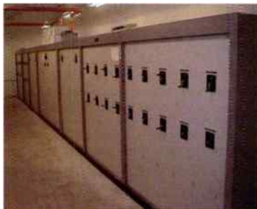
CUSTOM PHASOR INSTALLATION
