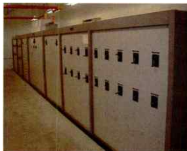
CUSTOM PHASOR INSTALLATION
