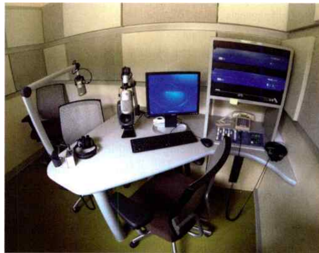
SAS Flush Mounted Cabinet with clock, hp amp and line inputs, Comrex DH20 Hybrid, Neumann BCM-104 mics, M!ka mic arms, Genelec 8010A monitor.
