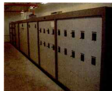
CUSTOM PHASOR INSTALLATION
