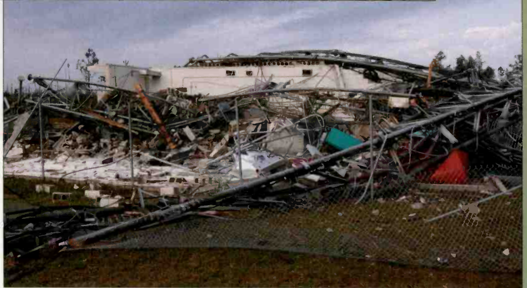
The tornado left mounds of debris in its wake
