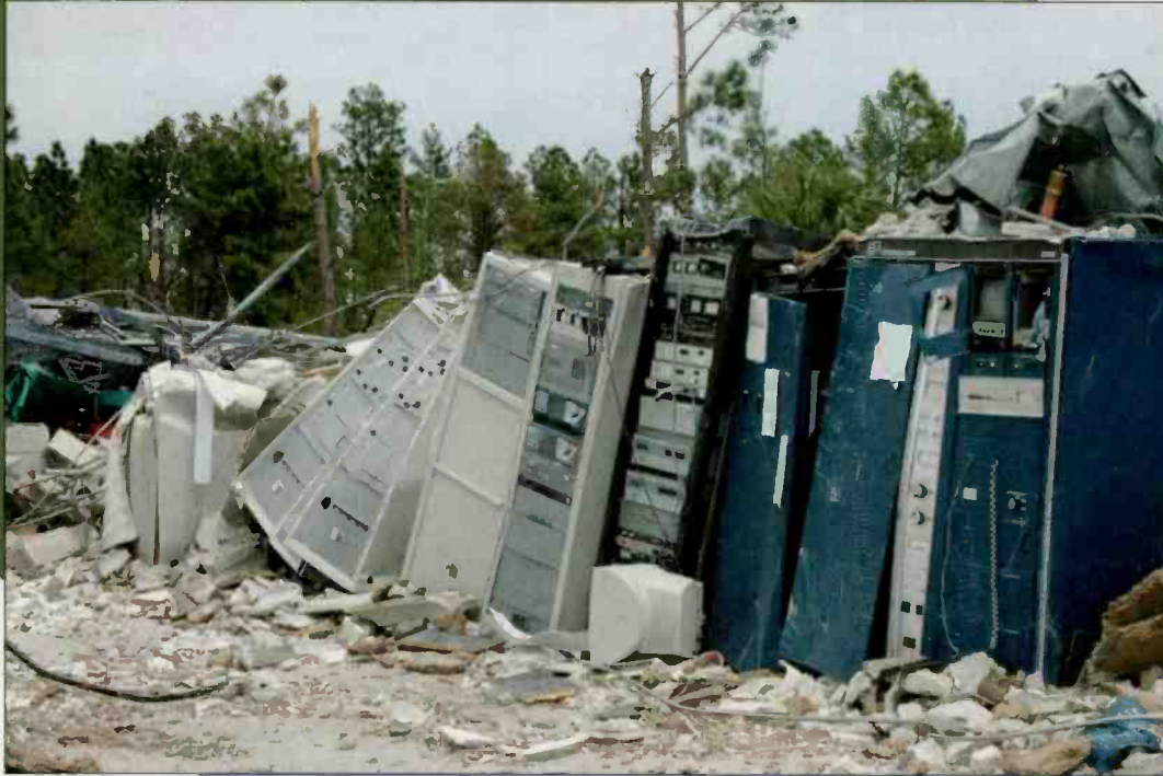
Damage to the racks
