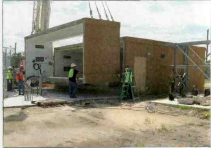
Assembling the prefabricated transmitter building
