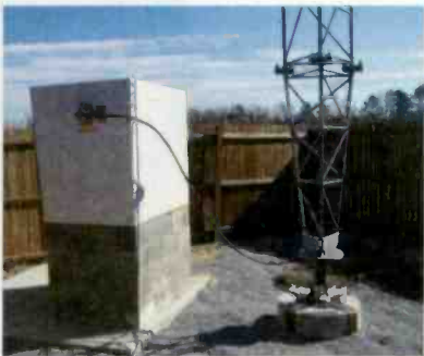
High-Power Antenna Tuning Units
