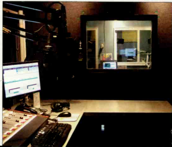
The door (just visible on the left) and window are now visible to the operator.
