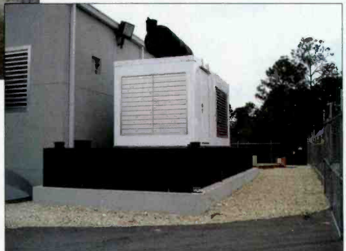
Above: A view of the old building with the new 40'x60' wing. Right: The Caterpillar 3412 diesel-power generator serves as backup for the new wing.
