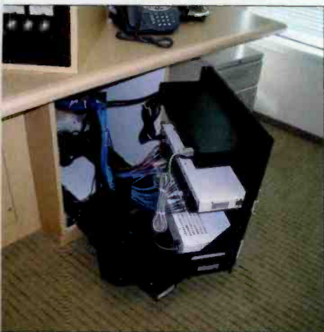
Pull-out mounts provide simplified front-of-rack access to equipment.
