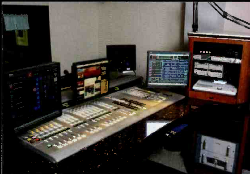
Control Room D, the control room for 790 the Ticket
