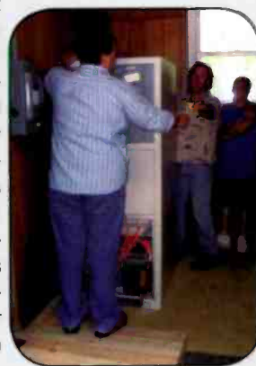
The hybrid transmitter is set into place.
