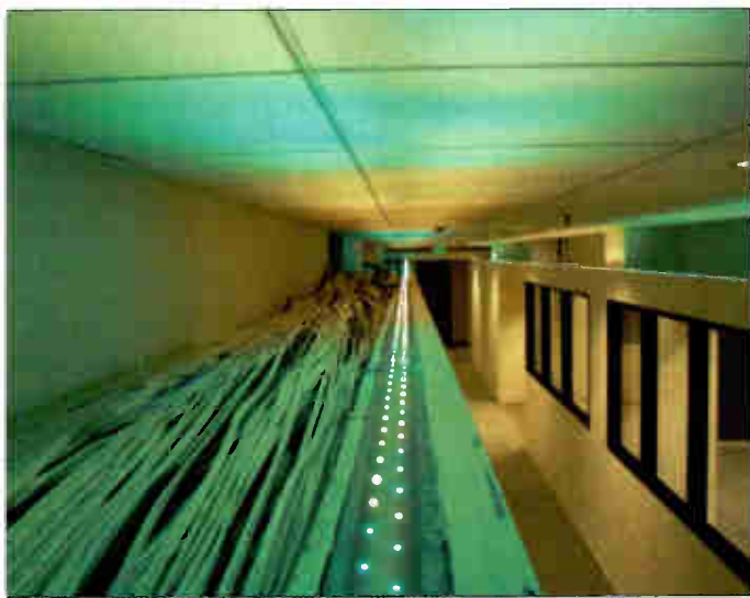
The corridor walls have an open space at the top that conceals the wiring trough. The designer used this space to provide colorful, indirect lighting, which provides a changing palette of colors.
