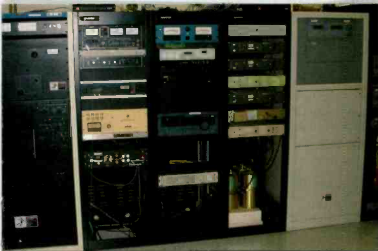
The WPYO split-level combining prototype using a Harris HT-5 and a Z-16HD transmitter. Above the center rack is the 3dB hybrid used for the combining of the outputs of the two transmitters.
