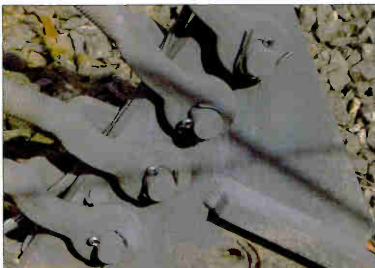
Stainless steel cotter pins are best. This anchor plate is cold galvanized for protection from rust.
