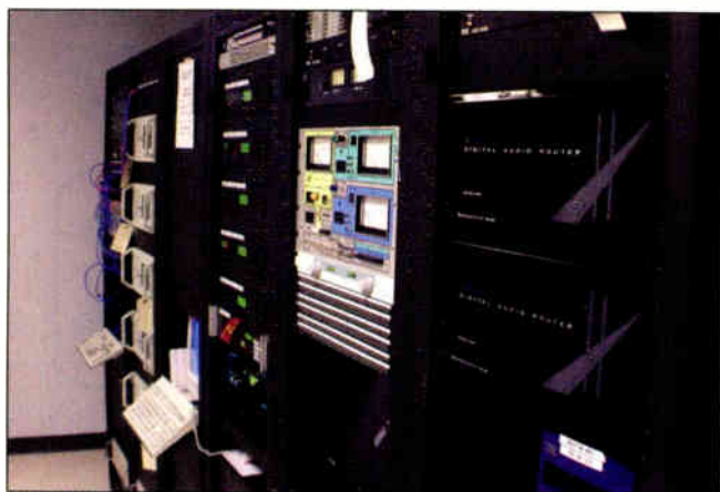
For audio distribution, Radio One chose the Wheatstone Bridge 2001 Digital Network router with redundant power supplies.
