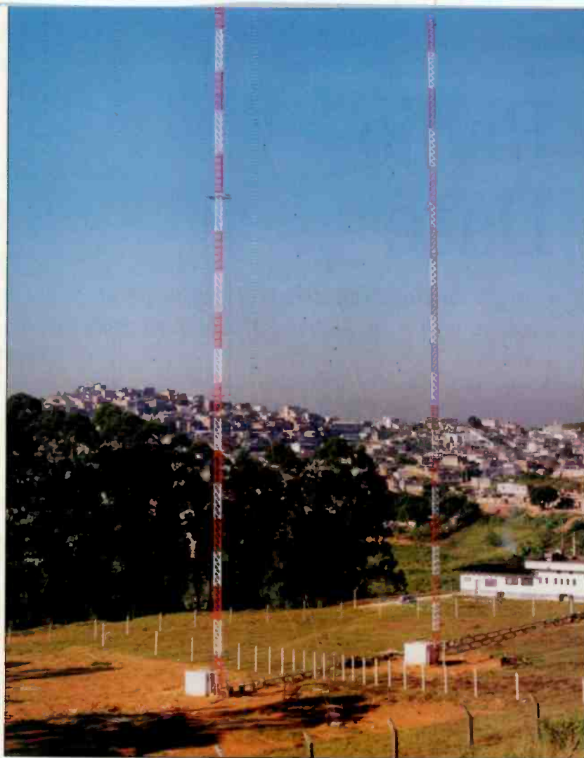
The two-tower array of ZYK-688. The tower on the left is the self-resonant folded unipole.
