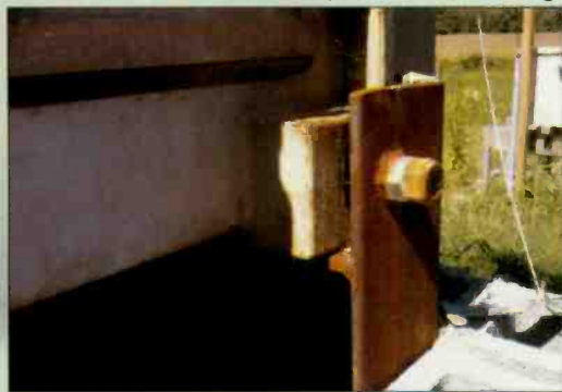
Detail of the corner showing the container stilts.
