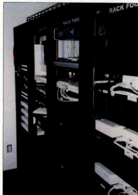
Most rack-room equipment can be externally accessed or controlled.
