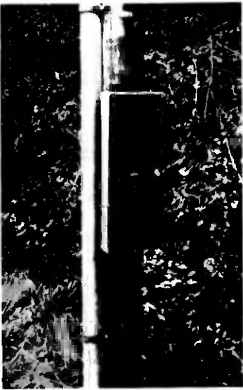
Fig. 18— SLC ™-40 pole-mounted repeater enclosure.
