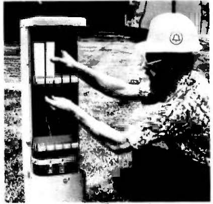
Fig. 19— SLC ™-40 pedestal-mounted repeater enclosure.
