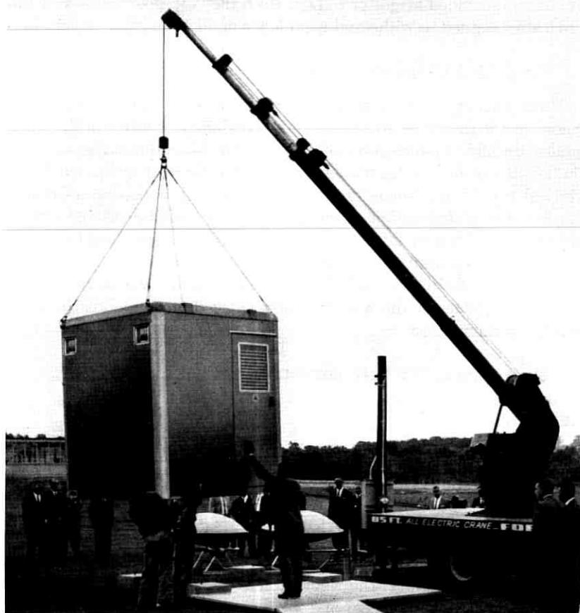
Fig. 42 — Installation of small shelter.
