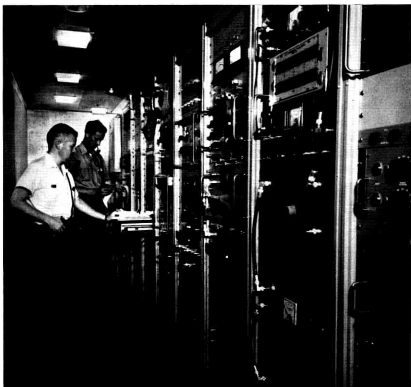
Fig. 4 — Interior view of telemetry van.
