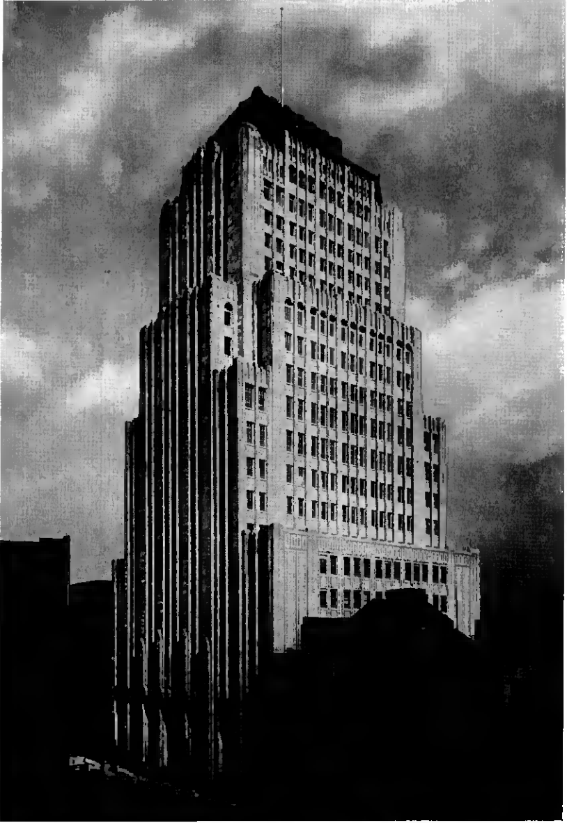
Fig. 24—Combined equipment and office building at Cleveland, Ohio containing headquarters of the Ohio Bell Telephone Company. 22 stories, 25,000 square meters of floor space. 13 floors designed for equipment including the toll board and ultimate dial equipment for 100,000 telephones. 9 floors arranged for office space.
