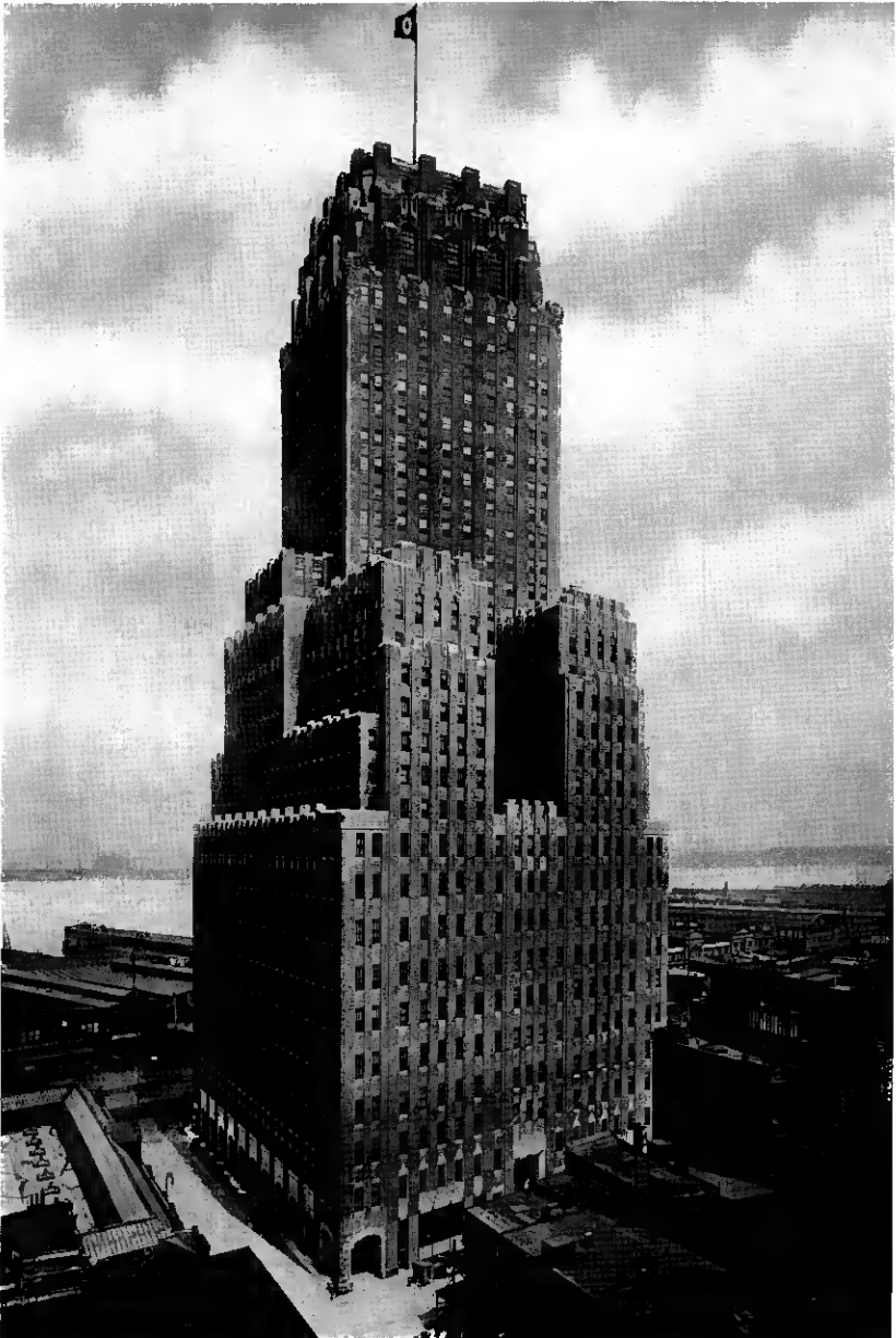
Fig. 22—Combined equipment and office building, New York City, containing headquarters of the New York Telephone Company, 31 stories, 66,000 square meters of floor space. Lower 9 floors arranged for toll tandem equipment and for dial equipment with an ultimate capacity of 100,000 telephones. Upper 22 floors arranged for offices with a capacity of about 5,000 people.
