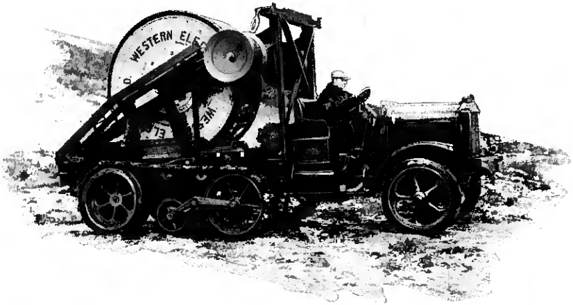
Fig. 50—Automobile truck equipped with tracks for hauling cable on private right of way. With tracks, speed about 16 kilometers per hour. Can carry 4500 kilogram reel up 40% grade. Tracks can be removed using special equipment provided for that purpose; without tracks speed 27 kilometers per hour.
