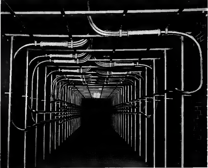
Fig. 14—Cable vault in Central Office, St. Louis, Missouri, showing entrance of cables through ducts and connecting to silk and cotton insulated cables extending up through the building.
