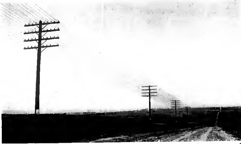
Fig. 38—Open wire pole line construction. Four 10-pin cross arms.
