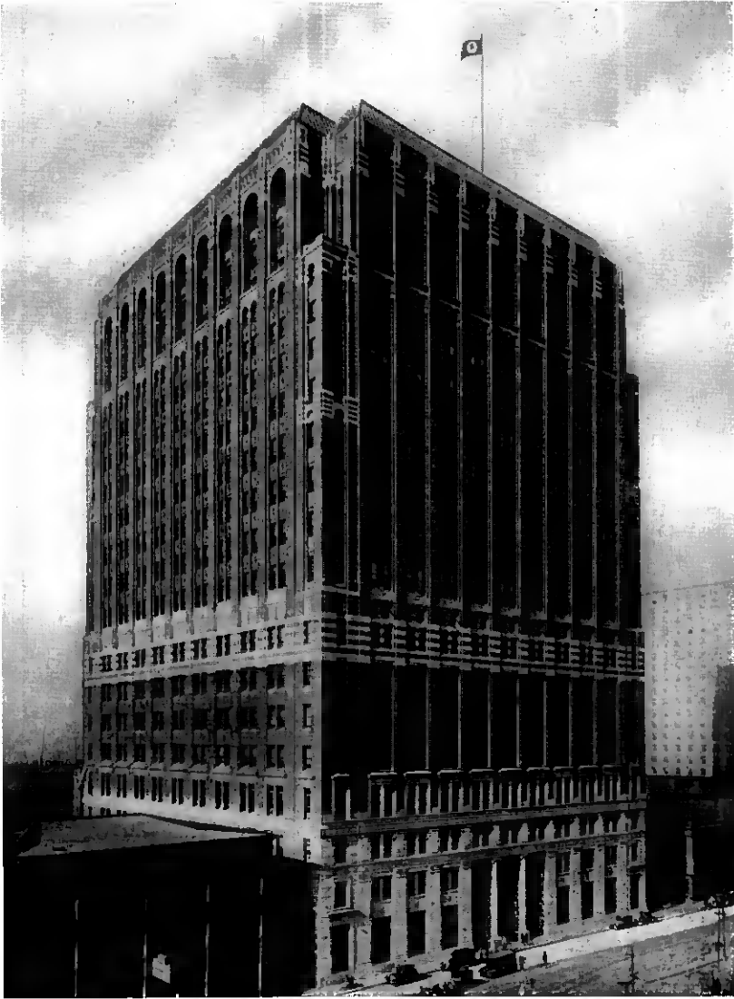
Fig. 23—Combined equipment and office building at Detroit, Michigan containing headquarters of the Michigan Bell Telephone Company. 19 stories, 28,000 square meters of floor space. 13 floors arranged for equipment including toll board and dial equipment to serve 60,000 telephones. 6 floors are arranged for offices.
