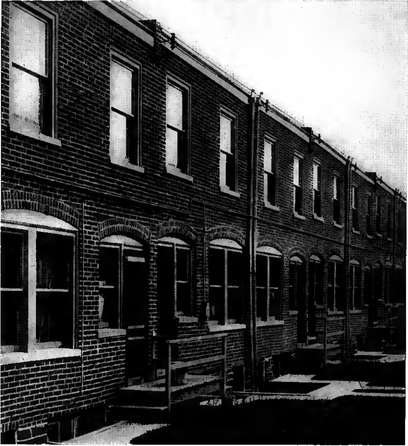
Fig. 12—Distribution telephone cable attached to rear wall of building showing terminal boxes and entrance by twisted pair into cellar.
