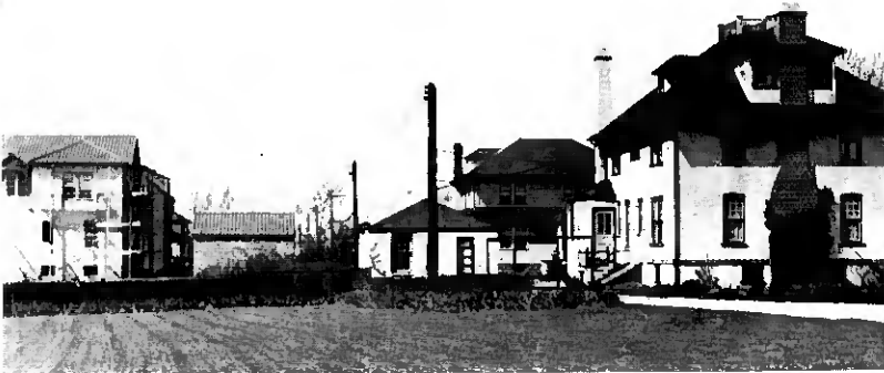
Fig. 11—Aerial cable distribution along rear property line. Poles used jointly for electric lighting power and telephone distribution.
