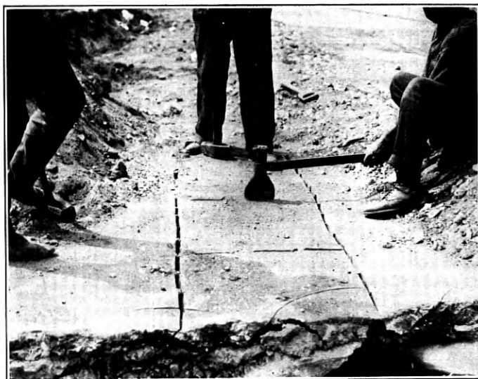
Fig. 24—Manual Method of Cutting Asphalt. Contrast with Fig. 22
