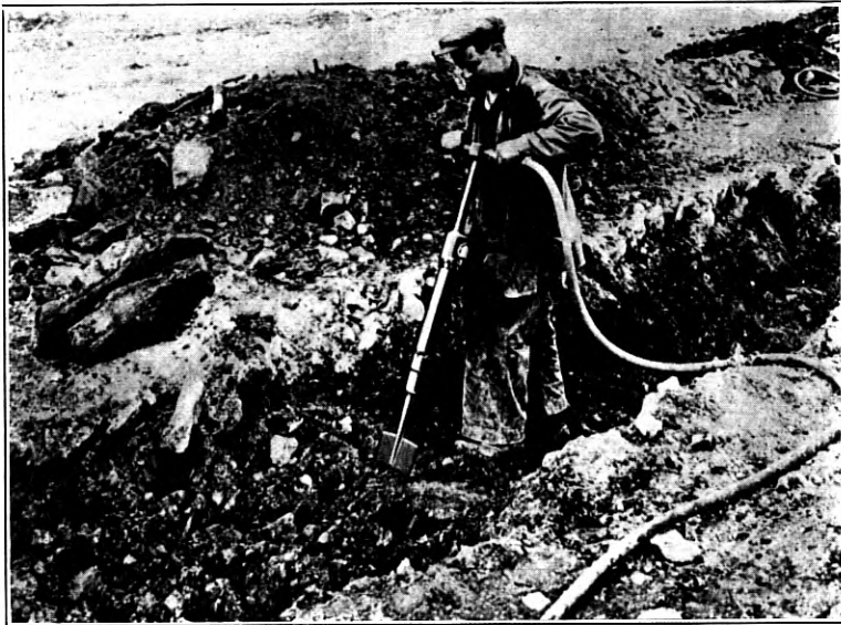
Fig. 25—Pneumatic Spade Replacing Hand Pick Method of Loosening Hard Soil
