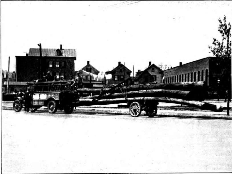
Fig. 11—Balanced Load of Chestnut Poles on Trailer
