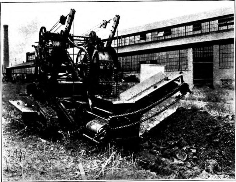
Fig. 16—Light Weight Trenching Machine.
