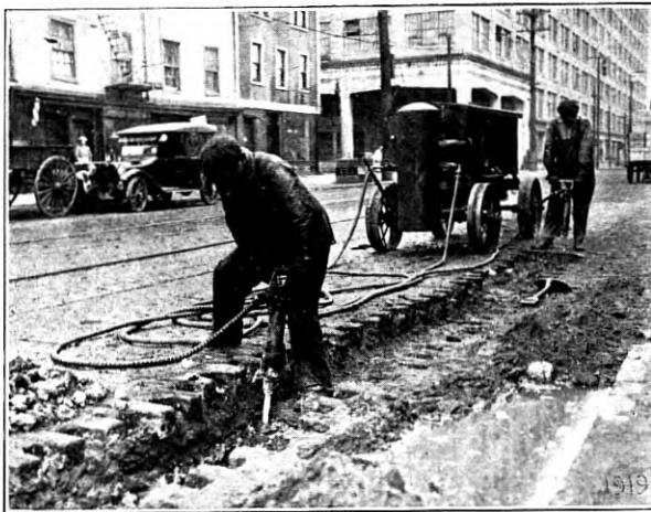
Fig. 21—Removing Granite Blocks and Breaking Concrete Base
