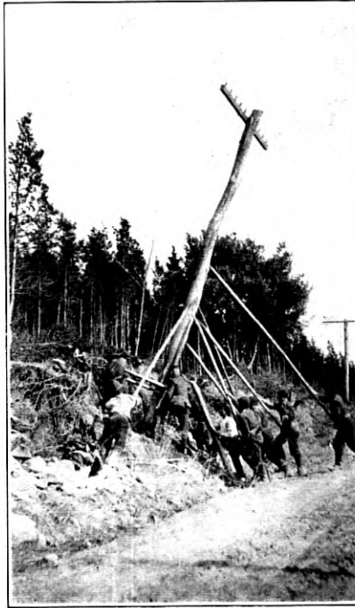
Fig. 6—Erecting Pole by Manual Methods. Contrast with Previous Operations
