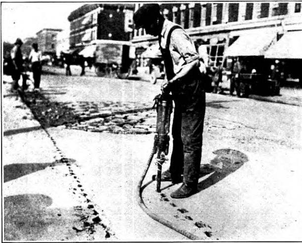
Fig. 22—Air Gun Cutting Asphalt
