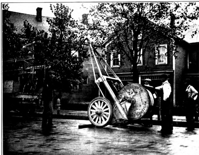
Fig. 9—Truck Being Used to Load Reel of Cable on Trailer
